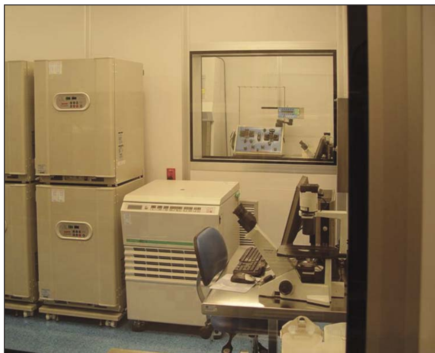
FIGURE 4. View of cleanroom #2. Cleanroom #1 is visible through the window. Locating the incubators or a centrifuge next to the cleanroom exhaust grilles helps control the environment by extracting particles, aerosols, humidity, or any hazardous gases.
