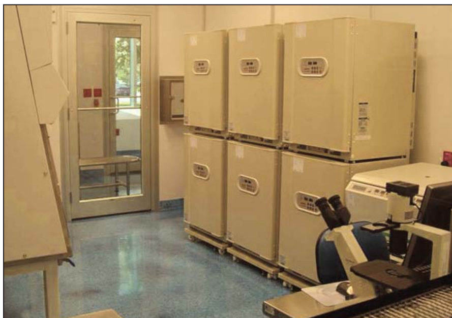
FIGURE 3. View of cleanroom #2.
